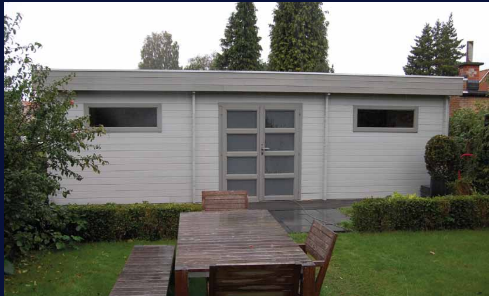
Mr Crawley chose a Moderna cinema room 9.0m x 3.0m in 45mm logs
